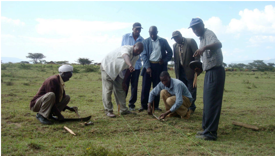
IDPs starting work on new plot. Pipeline, Nakuru district.
