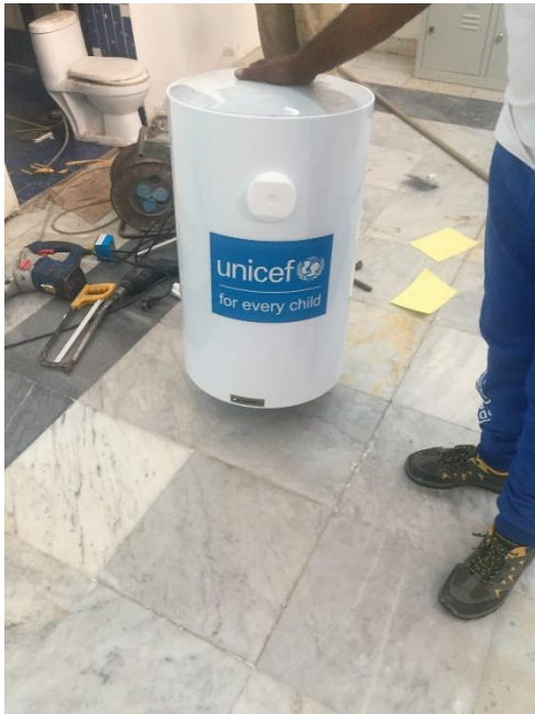
Rehabilitation of WASH facilities, Hay Elandalus collective shelter. Photo: UNICEF
