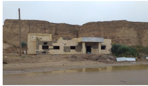
Health facility before rehabilitation
