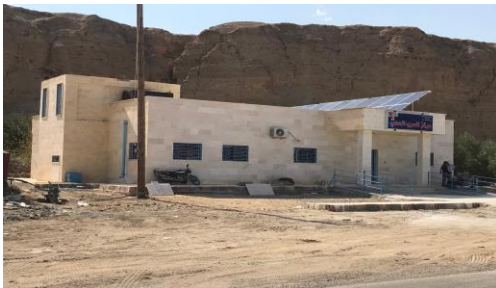
Health Facility after rehabilitation by Medair
